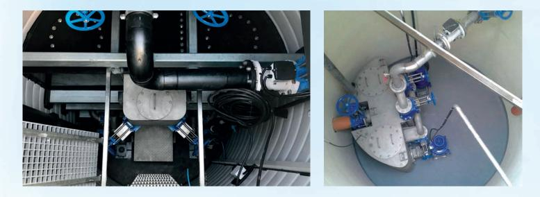
Dry well pumping stations are designed in a custom-made mode for each individual order.
