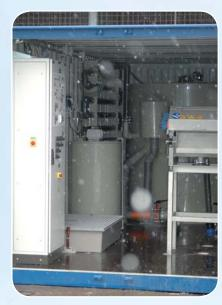
From the pumping station, wastewater is pumped over the mechanical pre-treatment section to the accumulation tank, where it is homogenised. From the accumulation tank, the water stream is uniformly pumped over the chemical treatment section to the flotation unit. After the chemicals are dosed in, pollutants partially tend to agglomerate (forming the socalled flocculi) that are separated in the flotation unit by air microbubbles and subsequently brought to the water surface as flotation foam.
