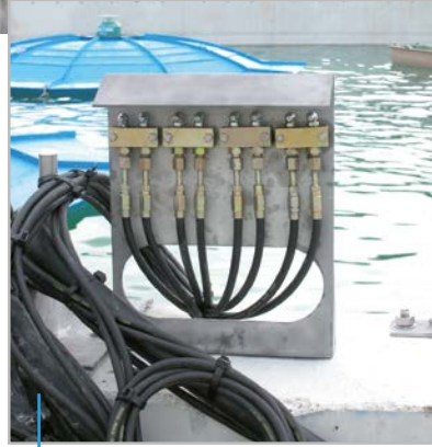
■ Motor with remote greasing & easy access greasing system
