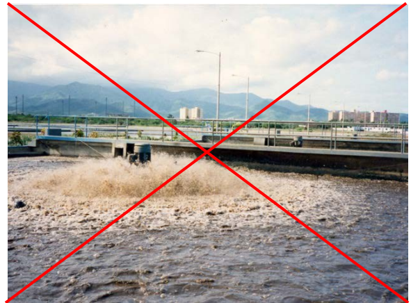
Excessive spray, aerosol, odor, and vapor draft.
